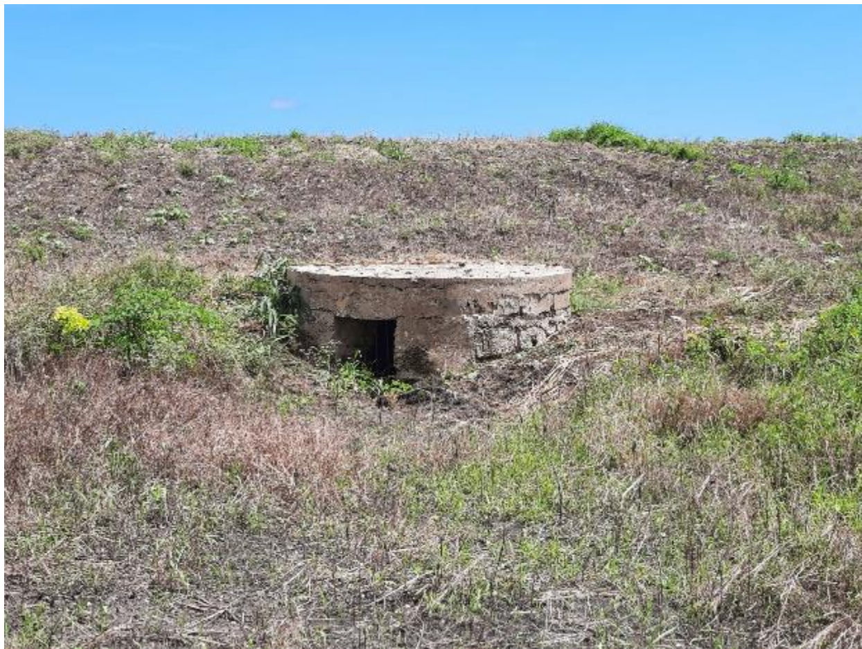
Photo 28 Drainage well H
