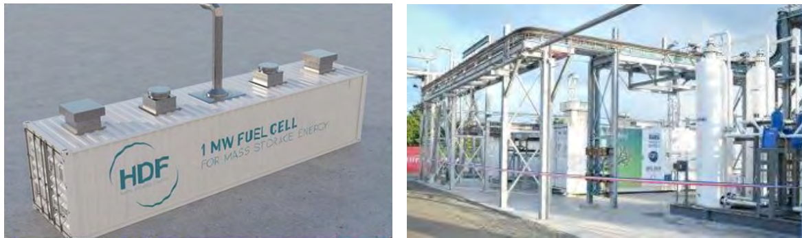
Figure 3.13 Examples of Containerised Fuel Cell (Left) and Containerised Fuel Cell System with Hydrogen Purification System (Right)
