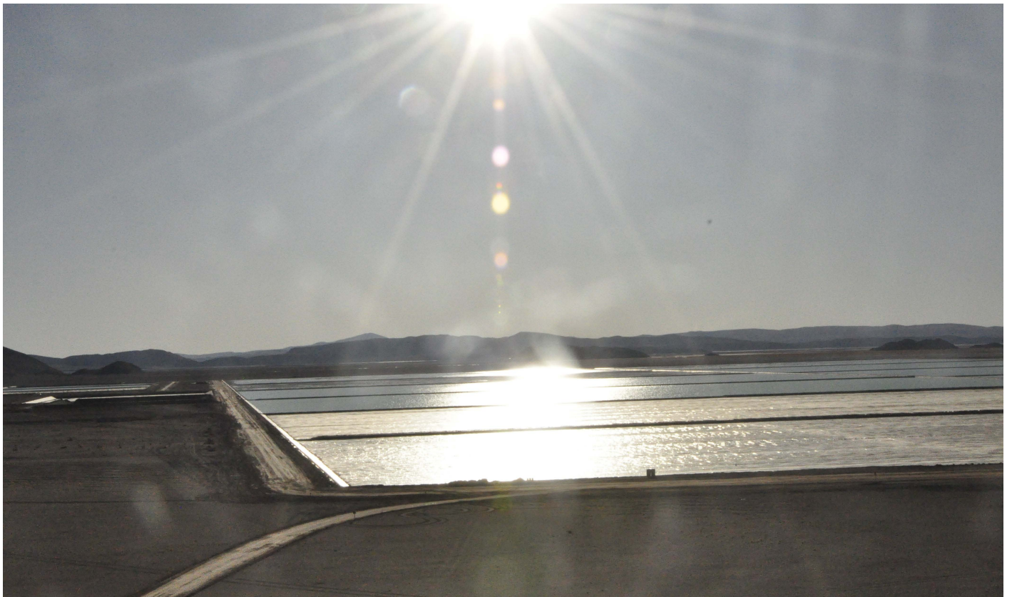
Ponds used to store and concentrate Lithium salt and solar radiation for brine evaporation.
