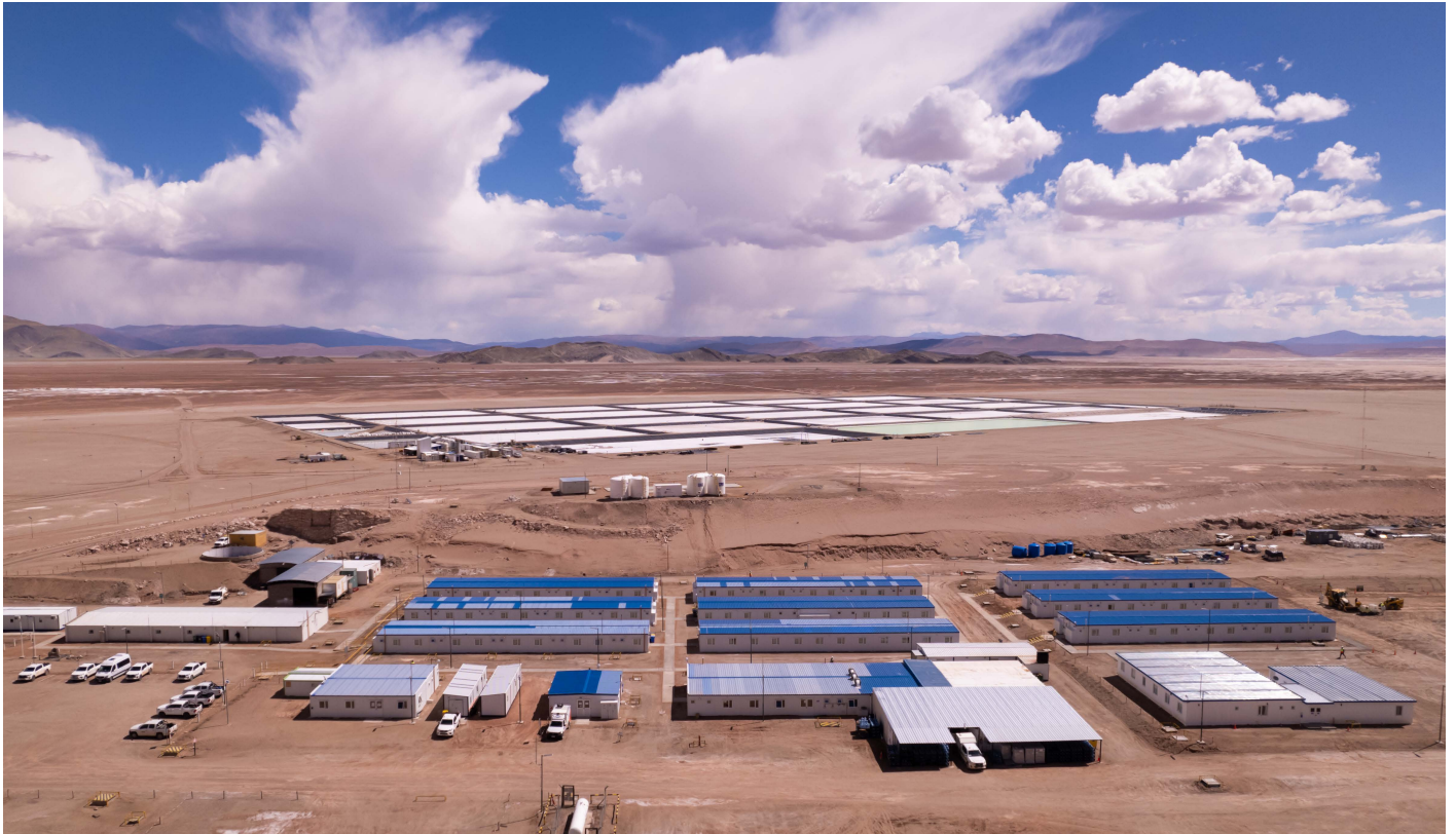
Sal de Vida Project infrastructure at project location.
