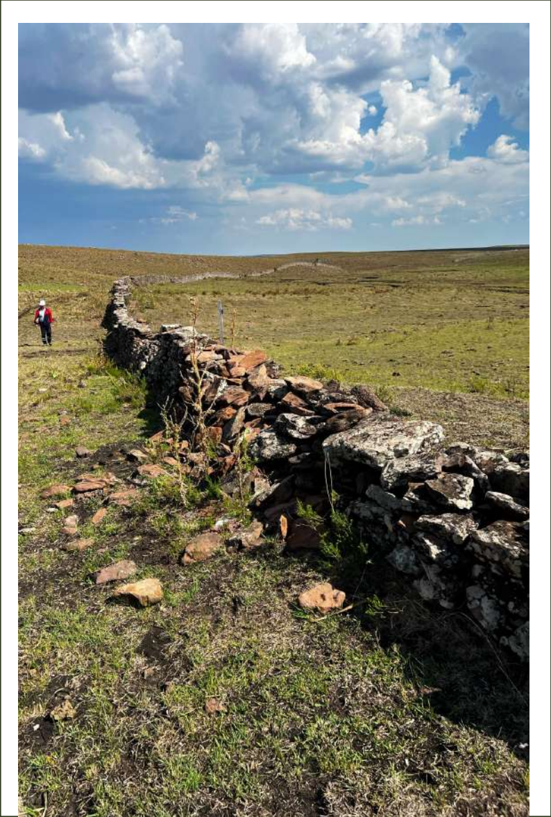
View of stone wall at Estancia Buen Retiro with several collapsed sections (most of them documented prior to project) with a section that had been reconstructed by farm workers in the foreground.
