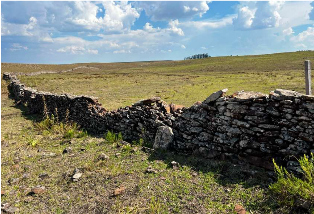
View of stone wall at Estancia Buen Retiro with collapsed sections. Note that the collapses occur with the same general section of the wall and that all of collapses point to one side opposite from the water drainage direction.
