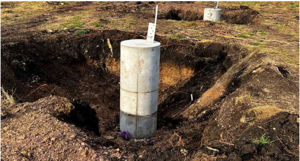
Construction of the foundation for a tower.
