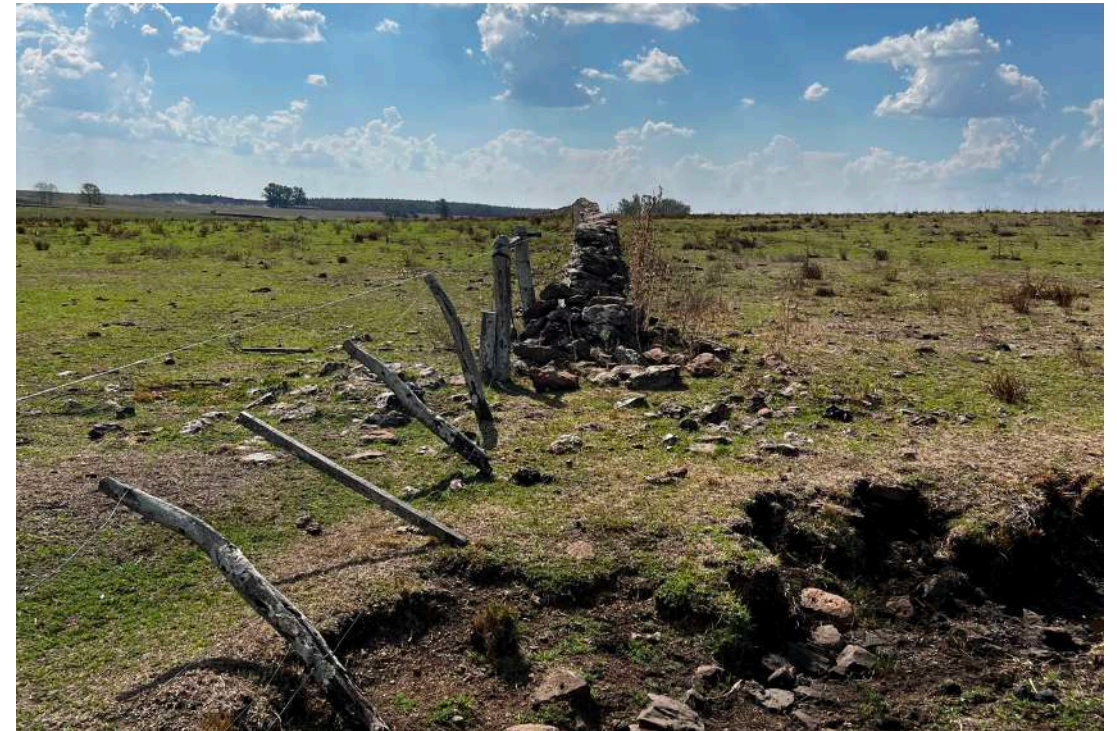
View of the one of the collapsed sections of the stone wall (documented collapse before the project ever started) at Estancia Buen Retiro. Note that the fence was installed over the stone wall foundation.
