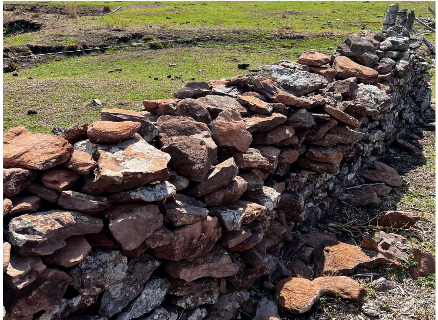
View of a section of the stone wall at Estancia Buen Retiro where the wall had previously been reconstructed by farm workers. Note the different color of the stones.
