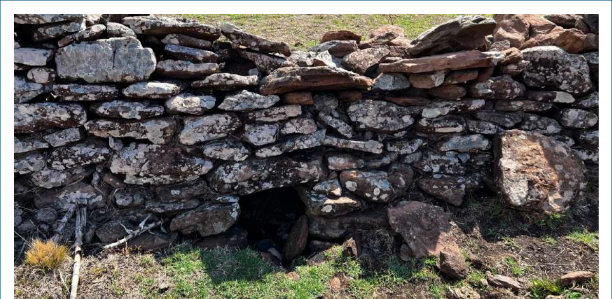
View of stone wall at Estancia Buen Retiro with drainage structure partially blocked.
