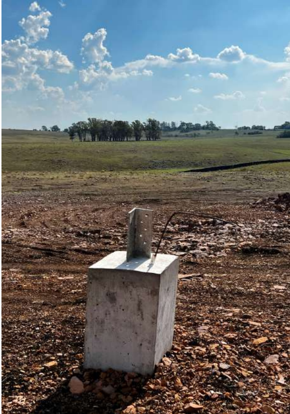
Construction of the foundation for a tower.
