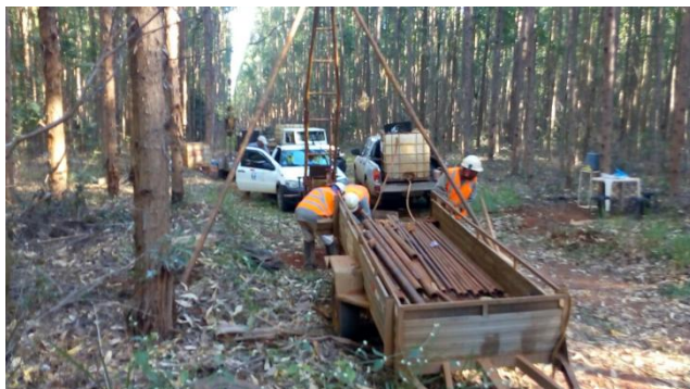
Figure 35 – SP02 Drilling hole. Source: GEOTORK, 2018.
