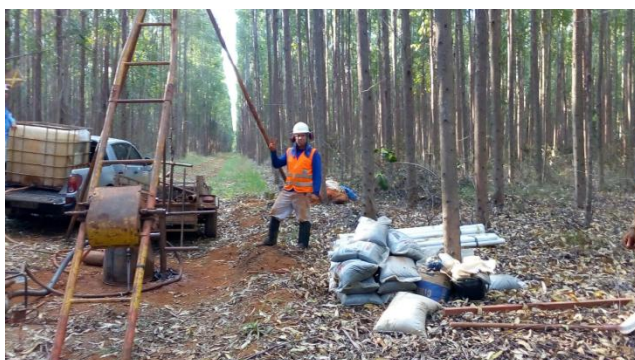
Figure 37 – SP04 Drilling hole. Source: GEOTORK, 2018.
