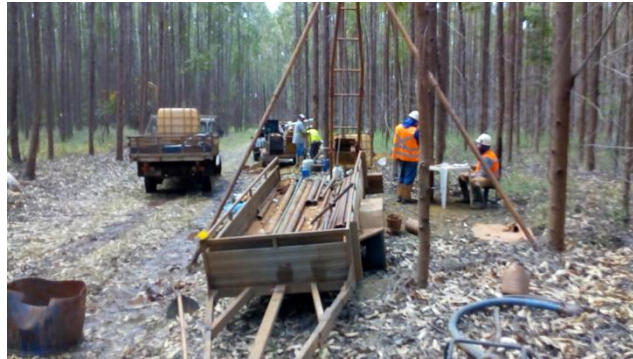
Figure 39 – SP06 Drilling hole. Source: GEOTORK, 2018.
