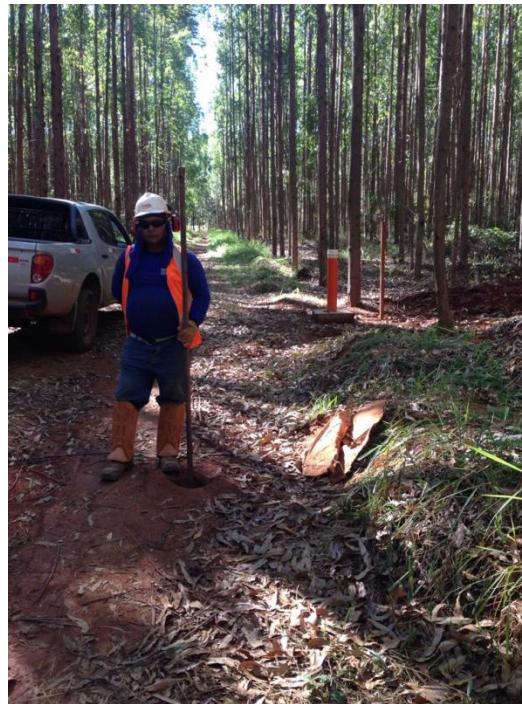
Figure 34 – SP01 Drilling hole. Source: GEOTORK, 2018.
