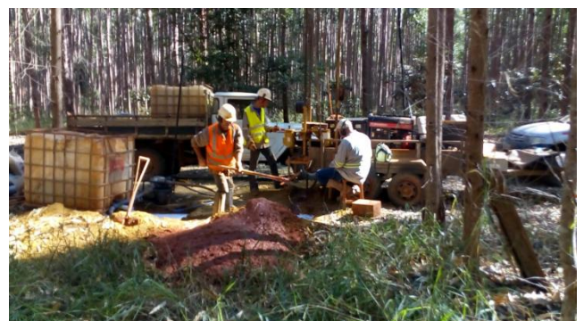
Figure 38 – SP05 Drilling hole. Source: GEOTORK, 2018.
