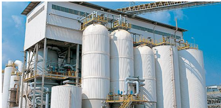
Figure 20 – Cooking Plant. Source: Pöyry, 2018
