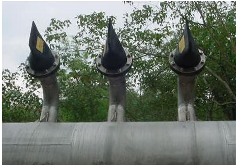
Figure 3 – Exemple of special check valve (duckbill type).
