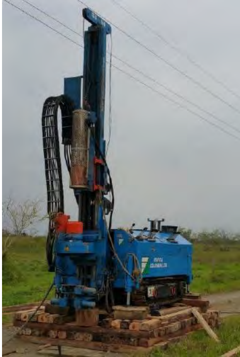
Photograph No. 2.2 Equipment for underground exploration of the ground Source: EDIFICA, 2015
