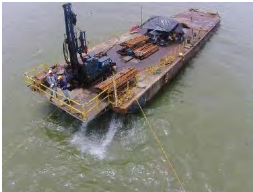
Photograph No. 2.1 Equipment for the exploration of the subsoil in water Source: EDIFICA, 2015
