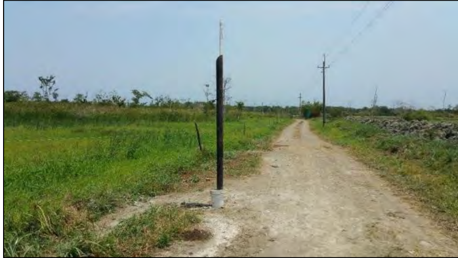
Photo 5.27 Piezometer installed on land. Source: EDIFICA COLOMBIA LTDA, in PIO S.A.S (2015) 170
