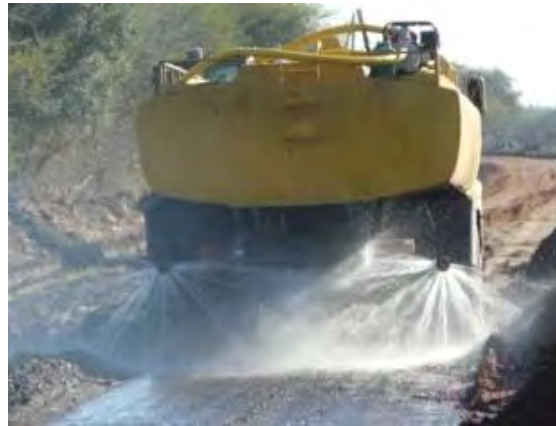
Photograph No. 11.1 Humidification of subgrade material when it is very dry Source: PIO SAS, September 2015.
