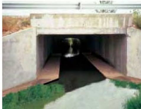
Figure No. 11.4 Examples of wildlife underpass structures Source: MMA - Madrid, 2006
