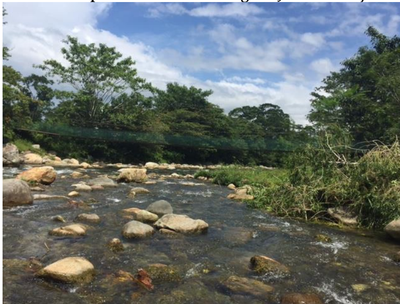
Photo 2 pedestrian access bridge to Jilamito Viejo
