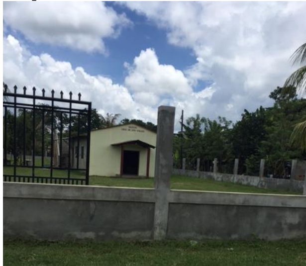
Photo 5 Improvement of church wall from Caserio El Retiro
