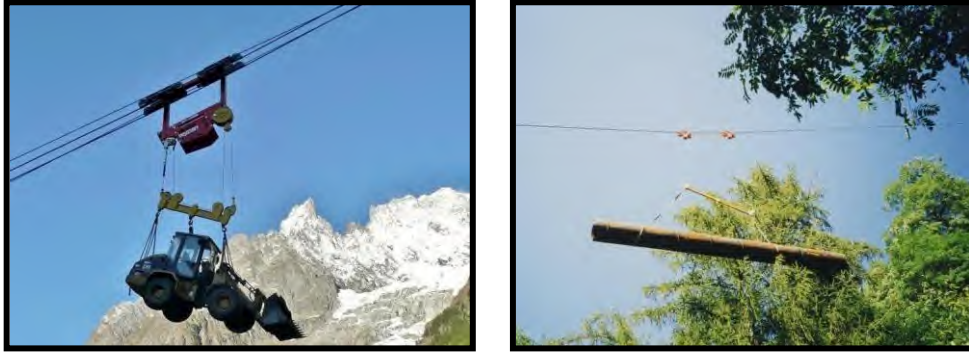
Example of cable car loading heavy machinery and steel pipes
