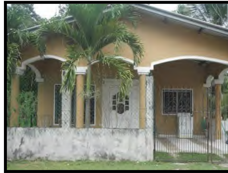
House for technical and administrative staff
