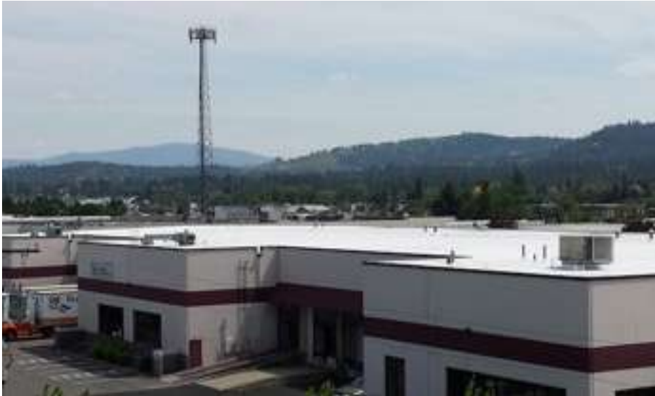
Figure 4.12 Concrete roof on SME, Eastern Washington, USA.
