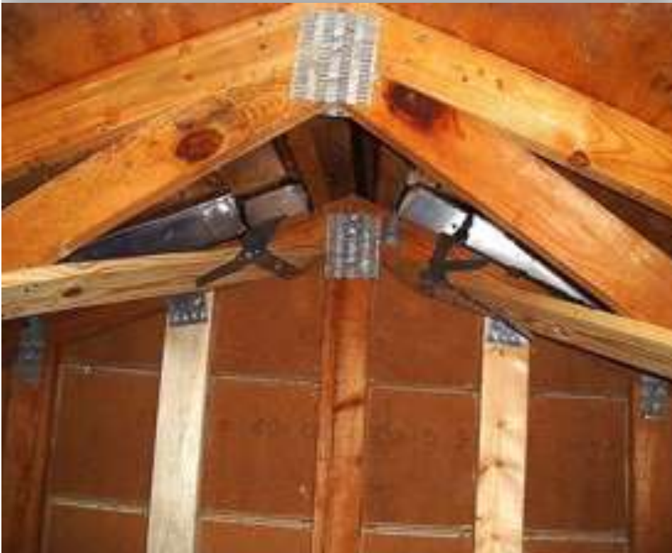
Figure 4.8 Examples of roof clips and ties.
