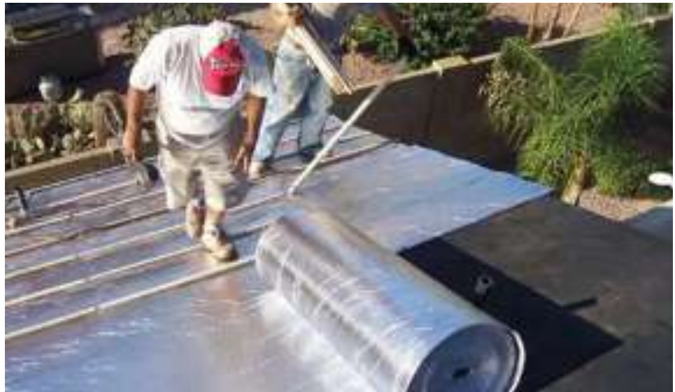
Figure 4.14 Example of radiant barriers to roof
