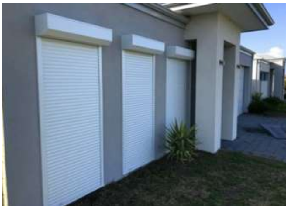
Figure R: Rolling Shutters installed on structure.
