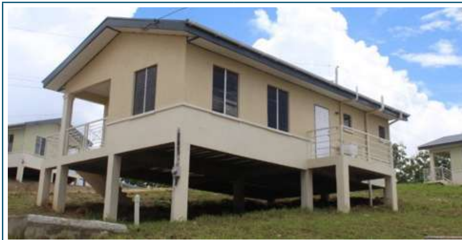
Figure H: Completed single story unit elevated on sloping site in Trinidad and Tobago
