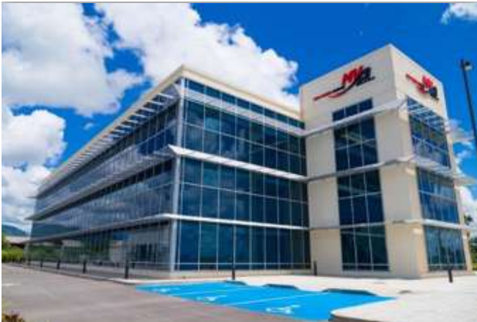
Figure 4.10 a) Glazing installed at Ministry of Works and Transport Office, Caroni, Trinidad and Tobago and b) Section of Impact Resistant Glazing.
