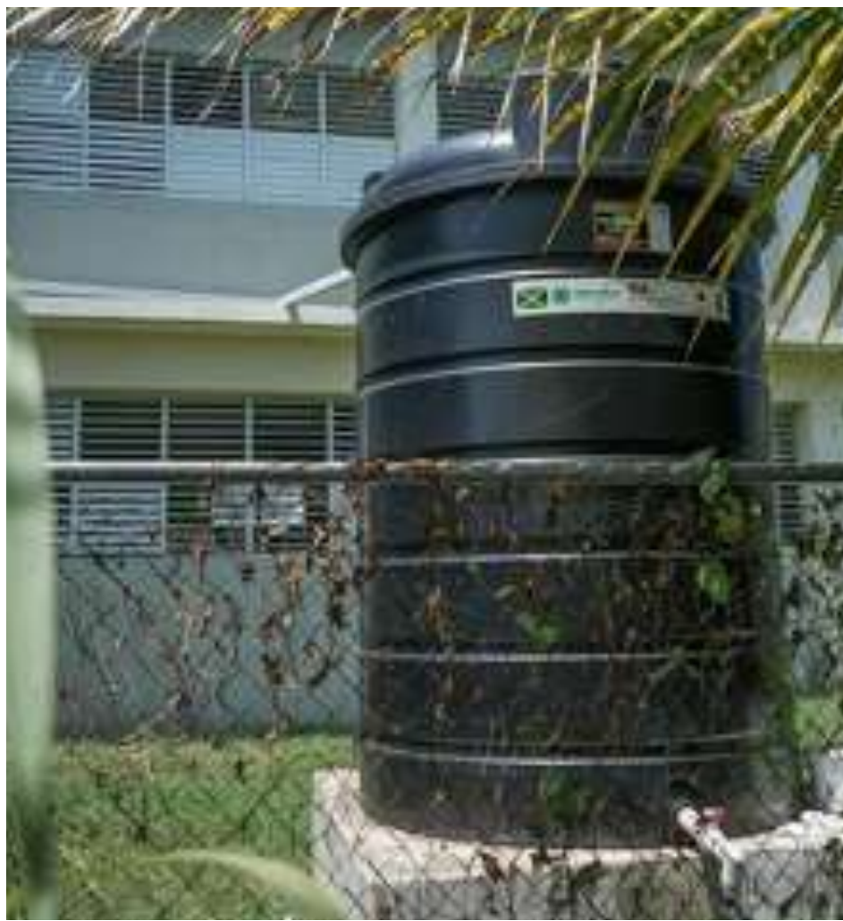
Figure N: Rainwater collection from a roof top in Jamaica.
