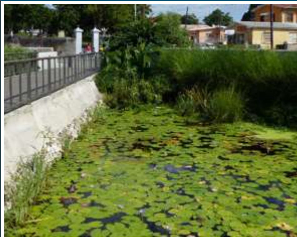
Figure L: Storm Water Retention Pond, Church Village Green, Bridgetown.
