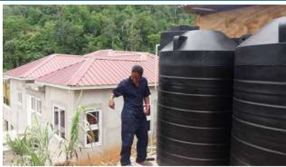
Figure BB: Water Storage Tanks
