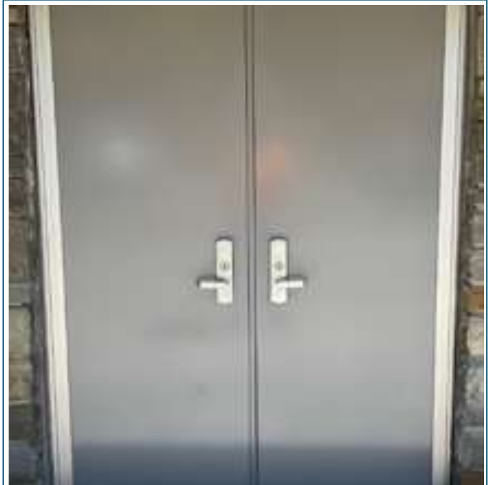
Figure I: Installation of flood door in New York, USA.
