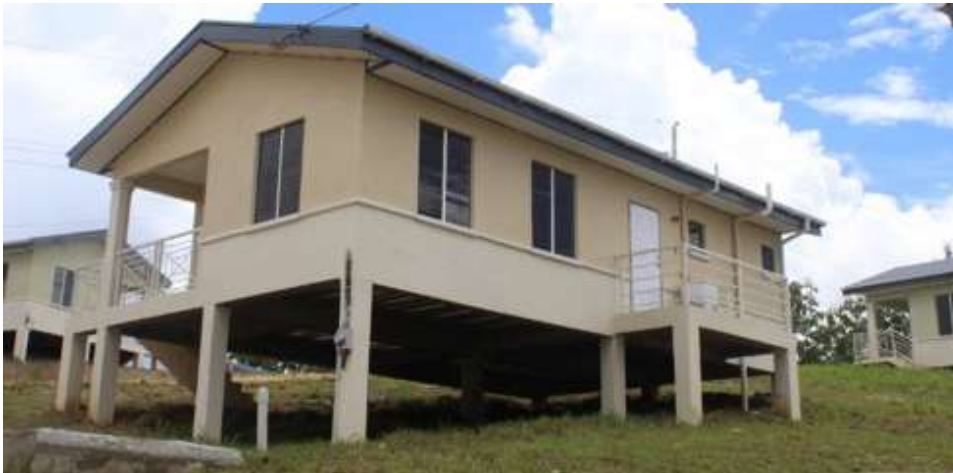
Figure 4.1 A completed single story unit of a 90-unit project in Trinidad and Tobago.
