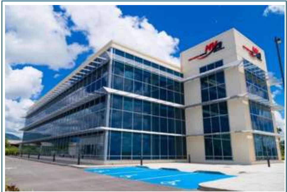
Figure Q: Glazing installed at Ministry of Works and Transport Office, Caroni, Trinidad and Tobago
