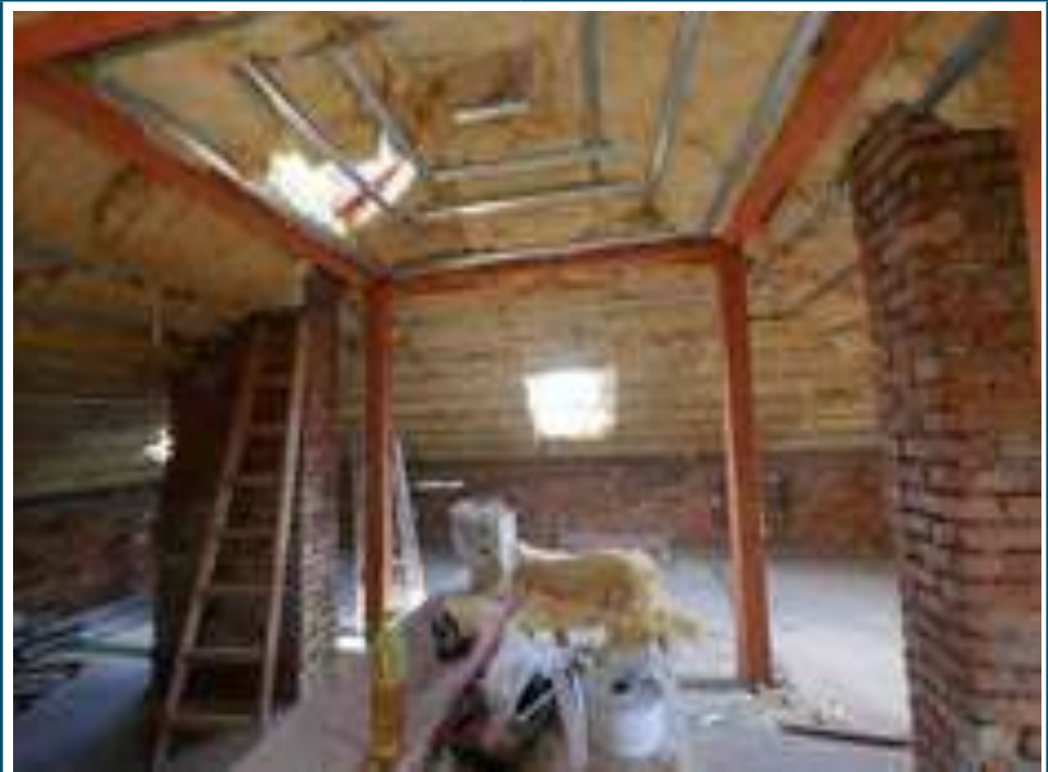
Figure U: Installation of the fiber installation on a concrete roof.
