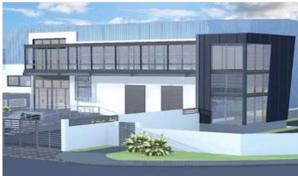
465 m2 warehouses for 50 to 100 employees with mezzanine floors, sandwich thermal insulation steel sheeting cladding
