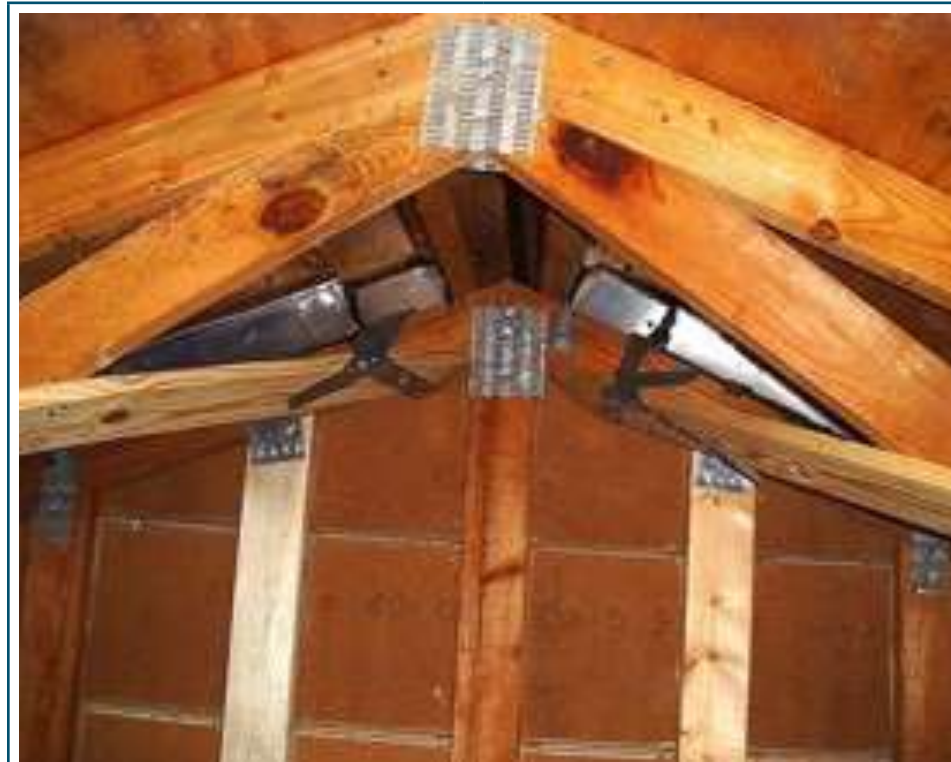
Figure O: Roof Clips and ties on a Timber Roof.
