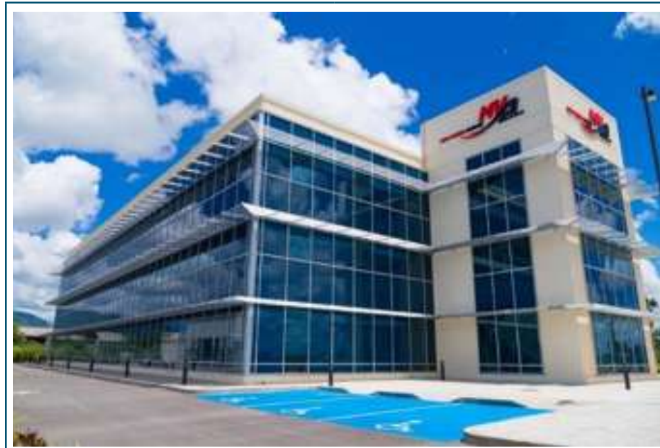
Figure Q: Glazing installed at Ministry of Works and Transport Office, Caroni, Trinidad and Tobago
