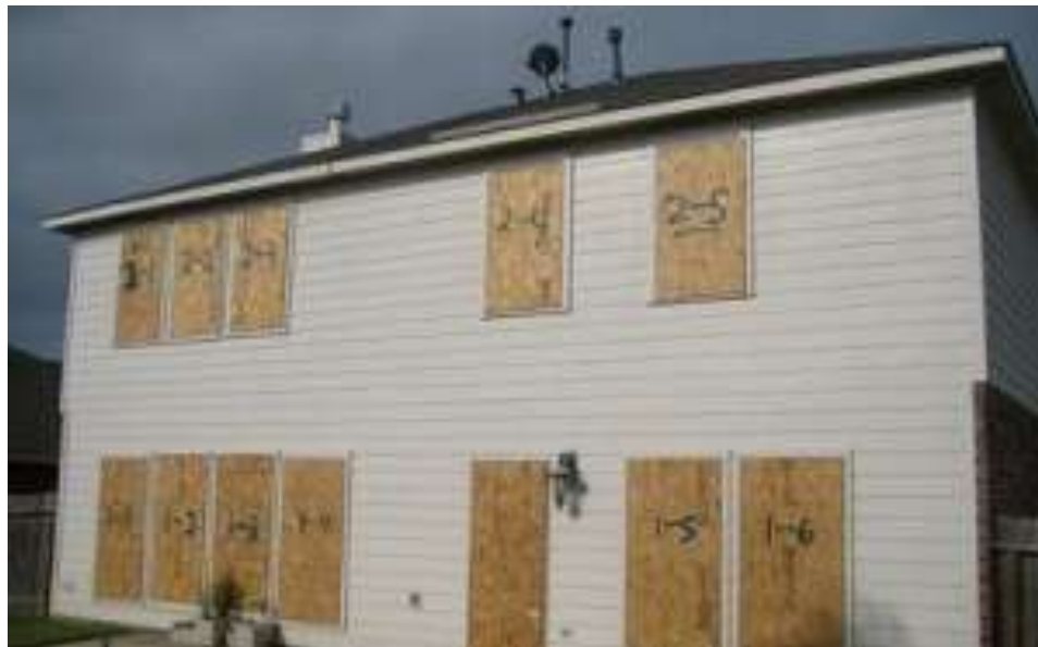
Figure 4.11 Timber shutter and Rolling shutters.
