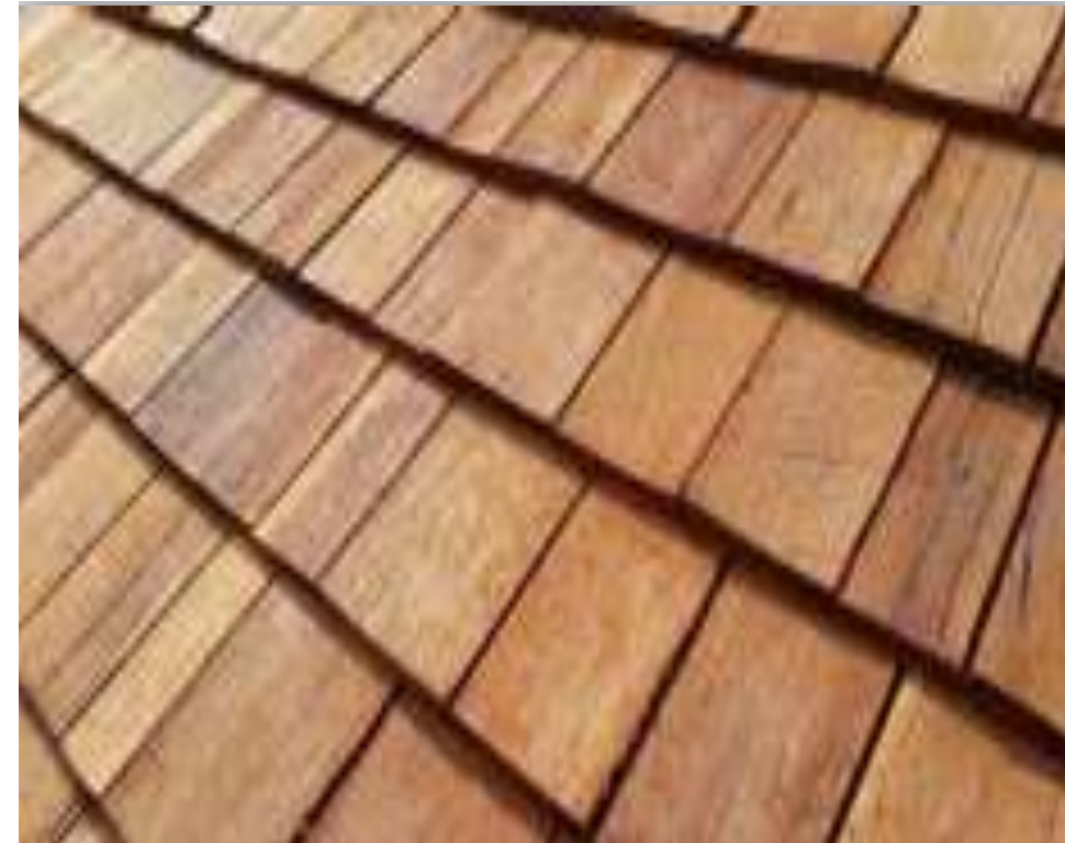
Using wooden roof tiles on 1/2" ply board in lieu of concrete roof. This would be coated with a waterproof sealant.
