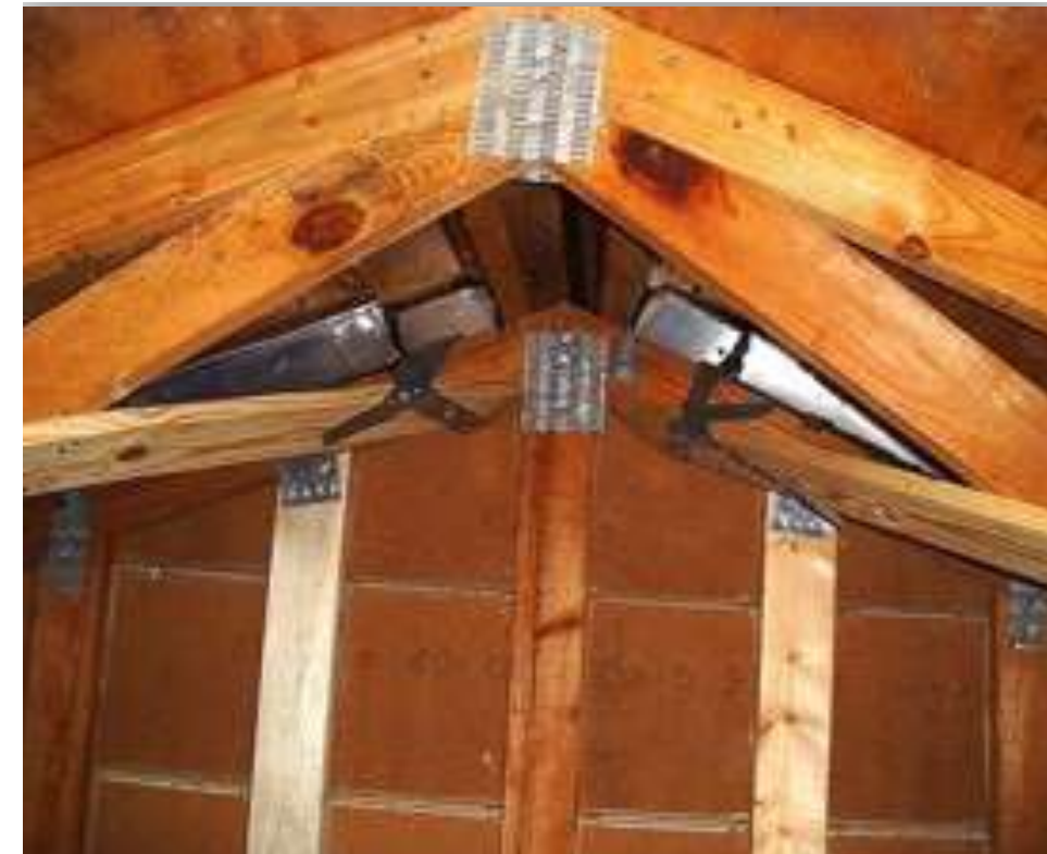
Figure 4.8 Examples of roof clips and ties.
