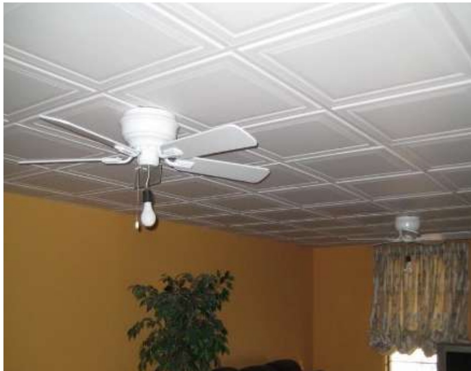
Using: a) sheet metal roof in lieu of a concrete roof and b) install a 1/2" insulative ceiling
