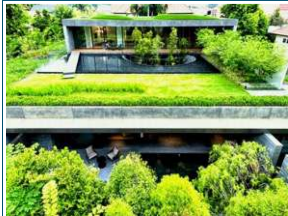
Figure M: Green Roof of a residential facility in Singapore.
