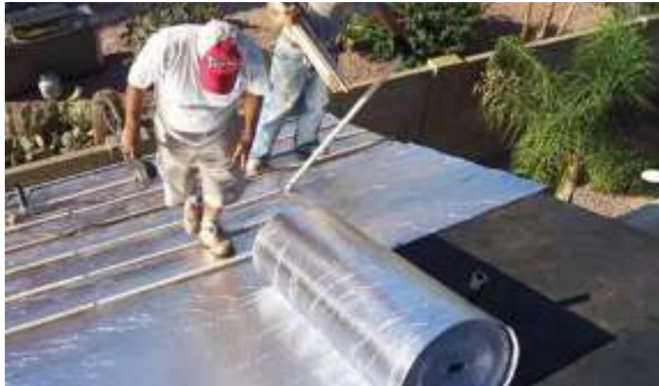
Figure 4.14 Example of radiant barriers to roof
