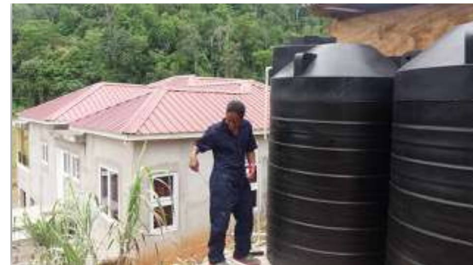
Figure 4.19 Example of water storage tank
