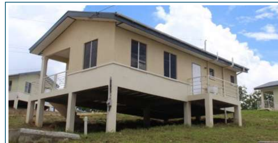
Figure H: Completed single story unit elevated on sloping site in Trinidad and Tobago
