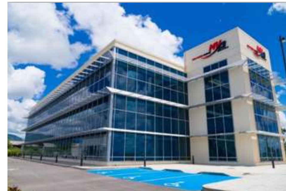
Figure 4.10 a) Glazing installed at Ministry of Works and Transport Office, Caroni, Trinidad and Tobago and b) Section of Impact Resistant Glazing.
