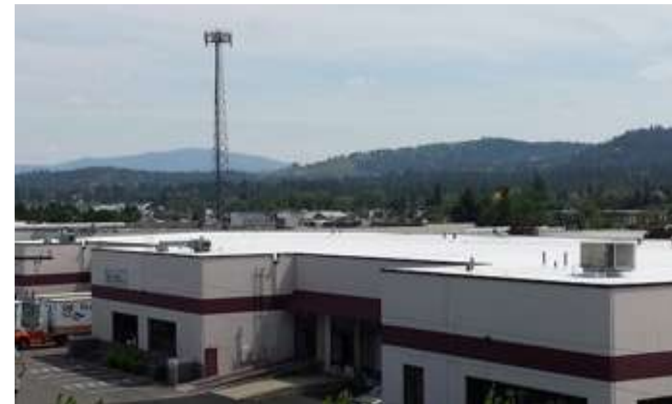
Figure 4.12 Concrete roof on SME, Eastern Washington, USA.
