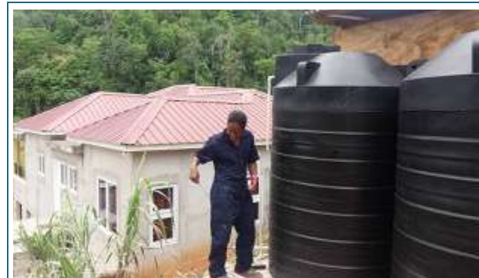
Figure BB: Water Storage Tanks
