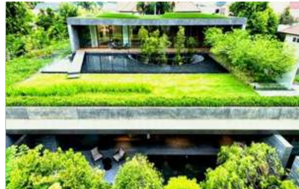
Figure 4.6 Examples of Green Roof atop: a) residential - Singapore and b) commercial building - Chicago, USA.
