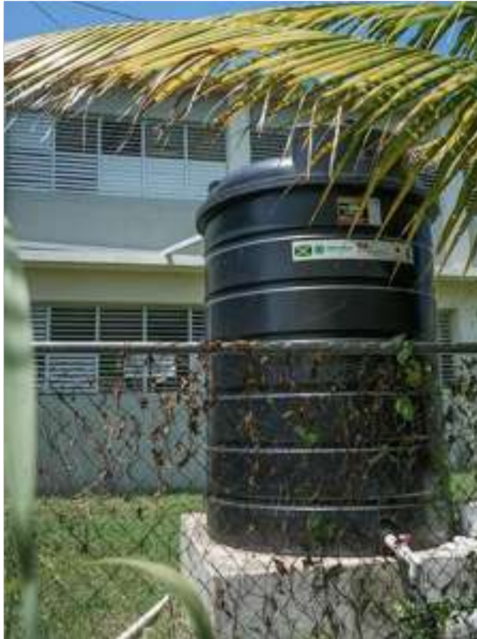
Figure 4.7 Rainwater collection from roof top, Jamaica.
