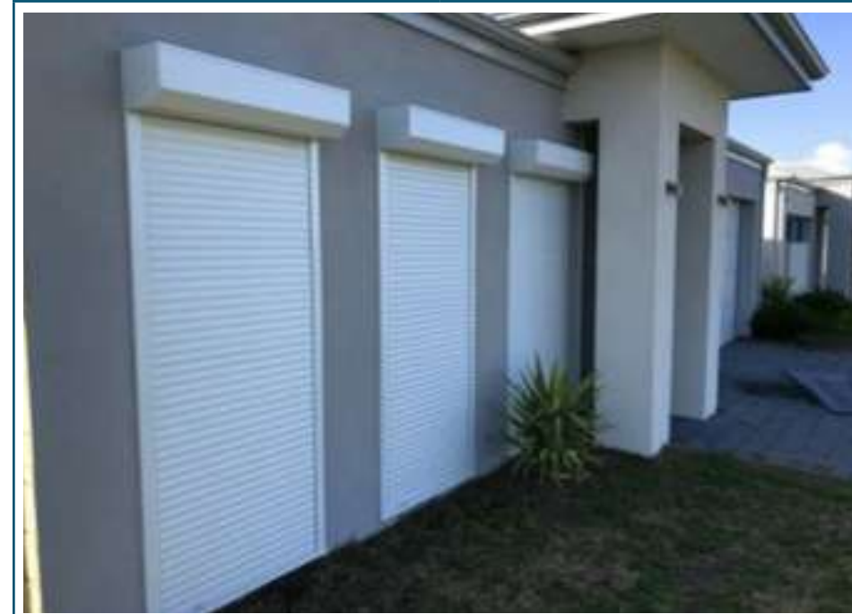
Figure R: Rolling Shutters installed on structure.
